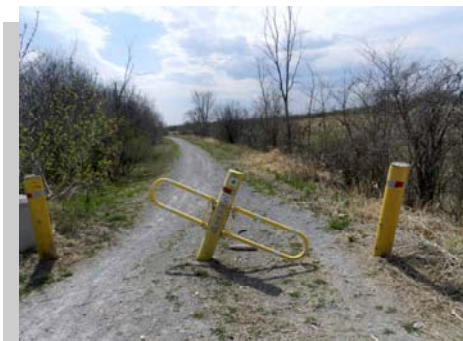
$700 damage to the gate at Acres Road.
